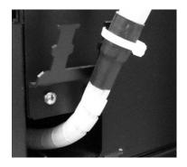
6. Secure feeder cable to cable entry clamp using supplied hose clamps or other suitable fastener like a zip-tie.
